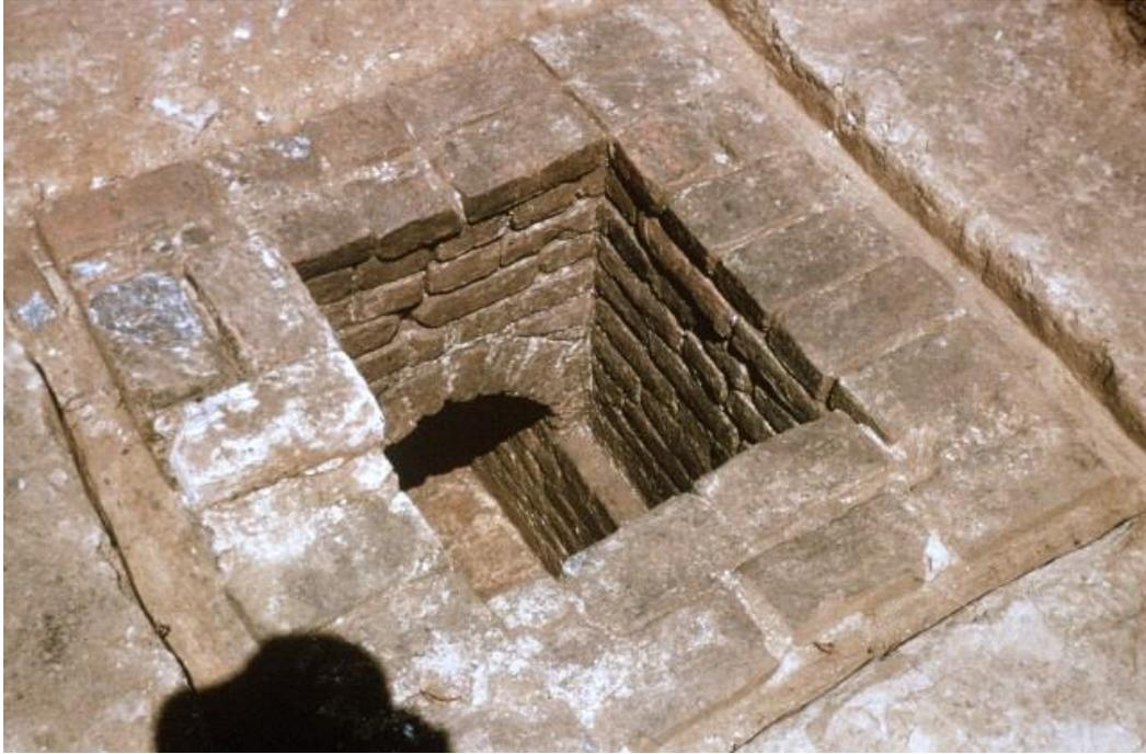
Figure 9: The manhole for cleaning out the drain.
