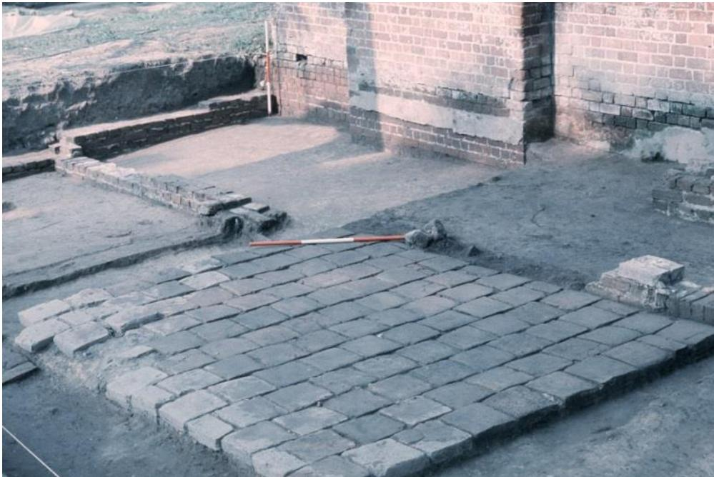
Figure 12: Brick pavers and remnant foundations of the early kitchen. Picture taken looking southwest, the east wall and chimney of the extant kitchen is in the background.
